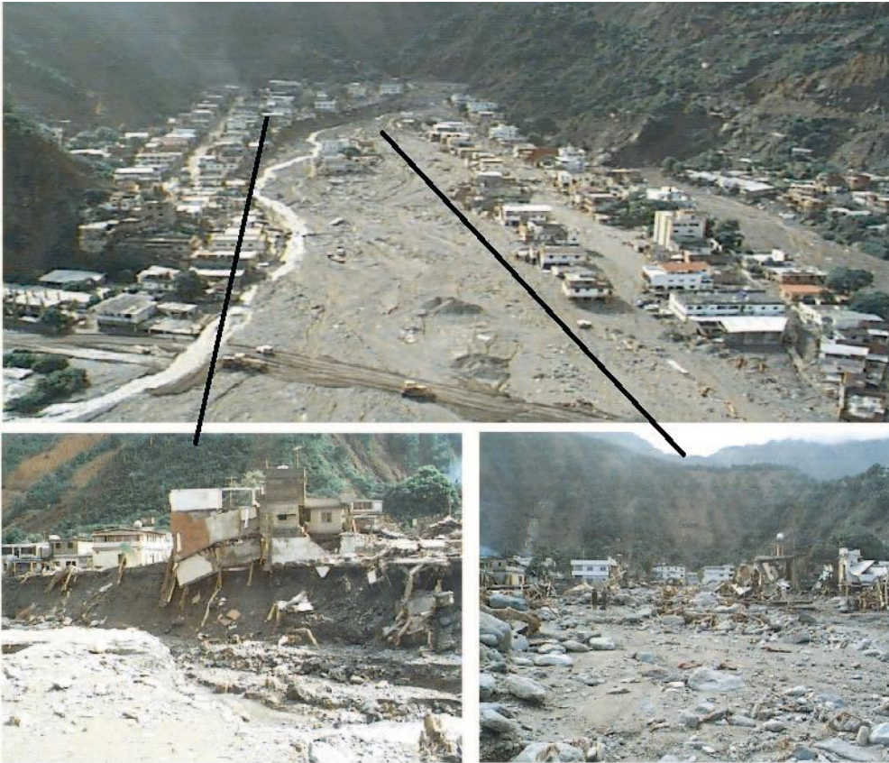
Figure 3. Aerial and ground views showing debris flow and flash flood damage at Carmen de Uria, January 2000.
