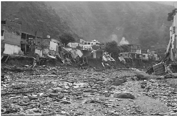
Figure 1. Homes destroyed by debris flow and flash floods, December 1999, Carmen de Uria, Venezuela.
